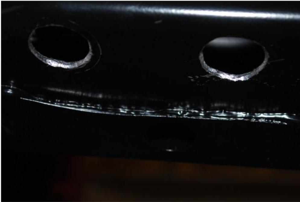
5. Using the 3/8" bit drill up through the 1" hole to enlarge the top holes. Repeat procedure for the other side.
